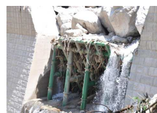
Fig.1 Steel open dam trapped rocks
