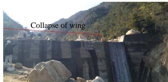
Figure 1 Collapse of concrete dam wing
