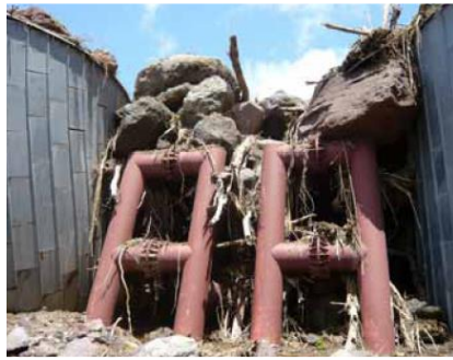
(a) Trapped rocks, wooden debris and sediment by steel open dam
