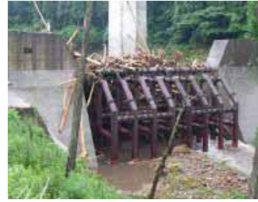
(a) Trapped wooden debris, rocks and sediment
