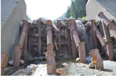
(b) Trapped large rocks; upper dam collapse.
