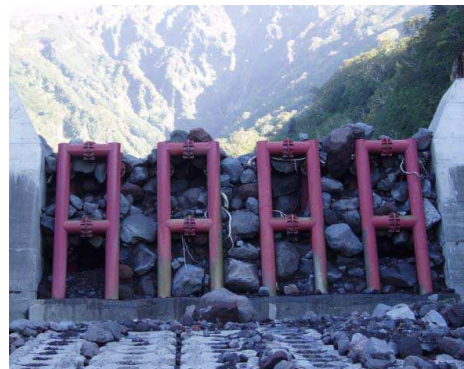
Fig.1 Only rocks trapped by a steel open dam
