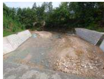
(c)最下流部の床固工の状況
