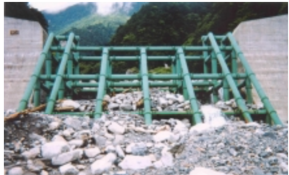
Fig.1 Open type steel check dam
