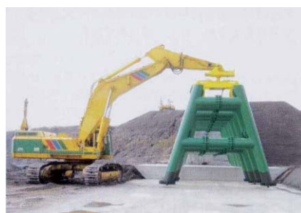
Photo 14: Transportation of Sabo dam
