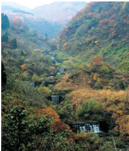
Photo 5 : Overall view of frame structure of Sabo dam
