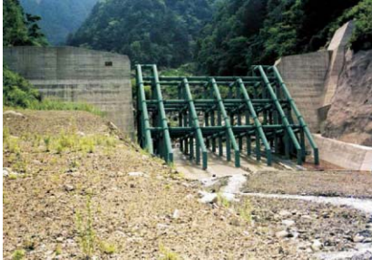
Photo 10: Status immediately after completion
