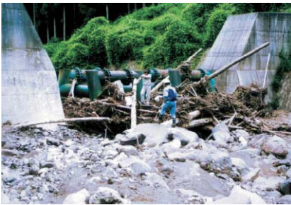
Photo 8 : Status of captured debris flow (upstream)
