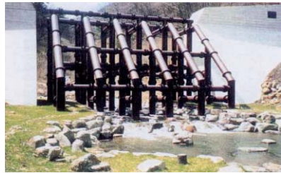
Photo 3 : Grid type steel Sabo dam
