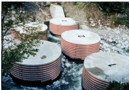
Photo 12: Status immediately after completion
