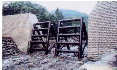
Photo 4 : Steel slit dam type L
