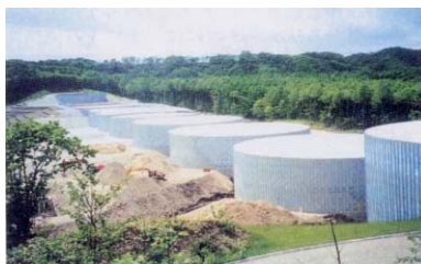
Photo 2 : Steel sheet pile dam
